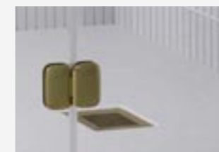
EXTERIOR VIEW OF HINGE
